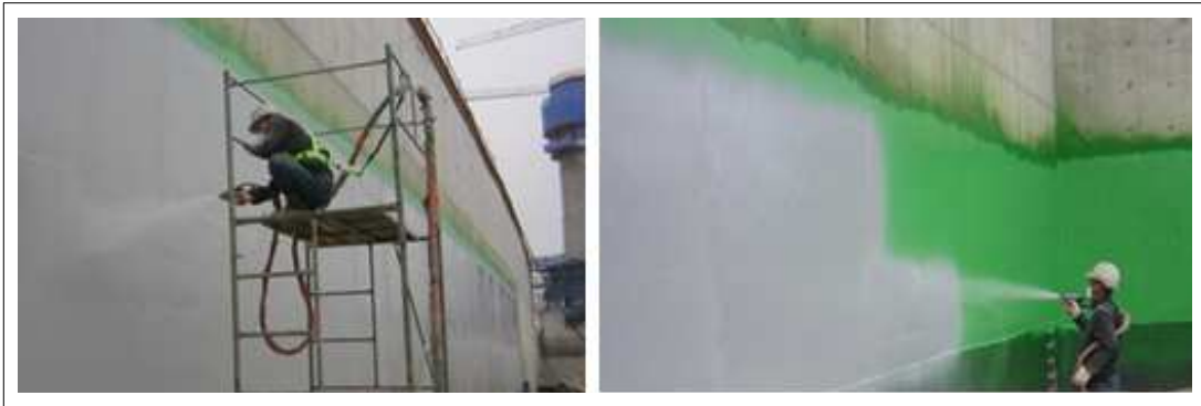
[KSC PU400 3rd 시공사진]
