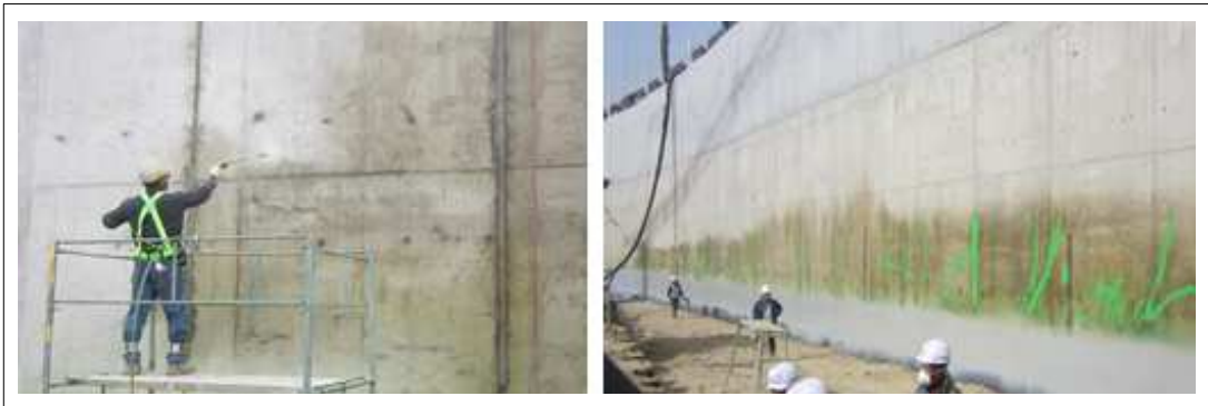
[KSC P100 1st 시공사진]
