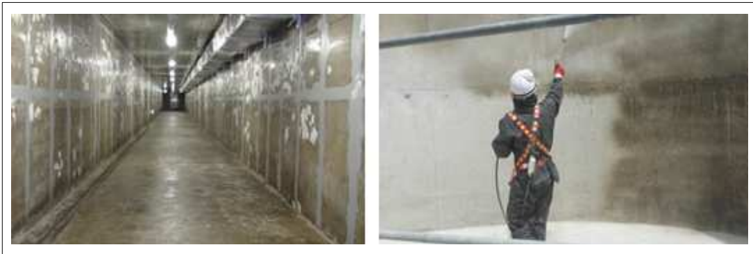
[KSC P100 1st 시공사진]
