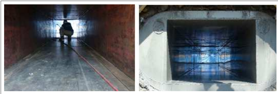
[KSC SP100 1st 시공사진]
