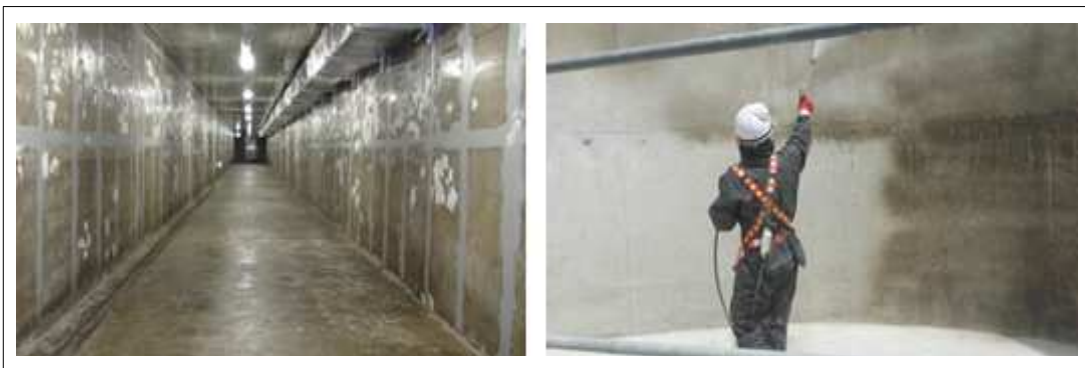
[KSC P100 1st 시공사진]
