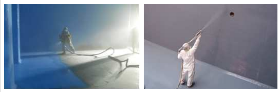
[KSC PU200 3rd 시공사진]
