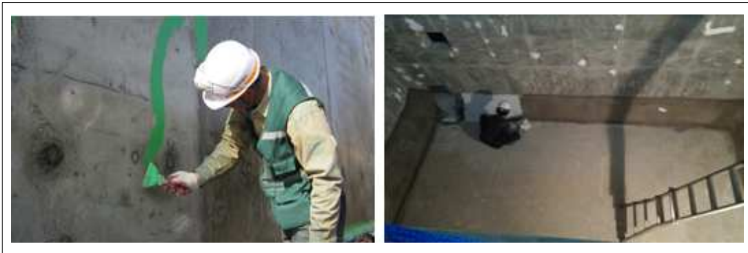
[KSC P100 1st 시공사진]
