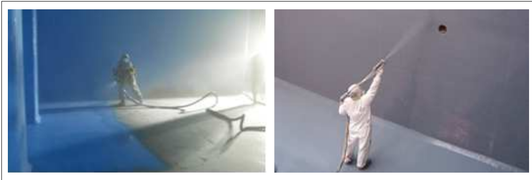
[KSC PU200 3rd 시공사진]
