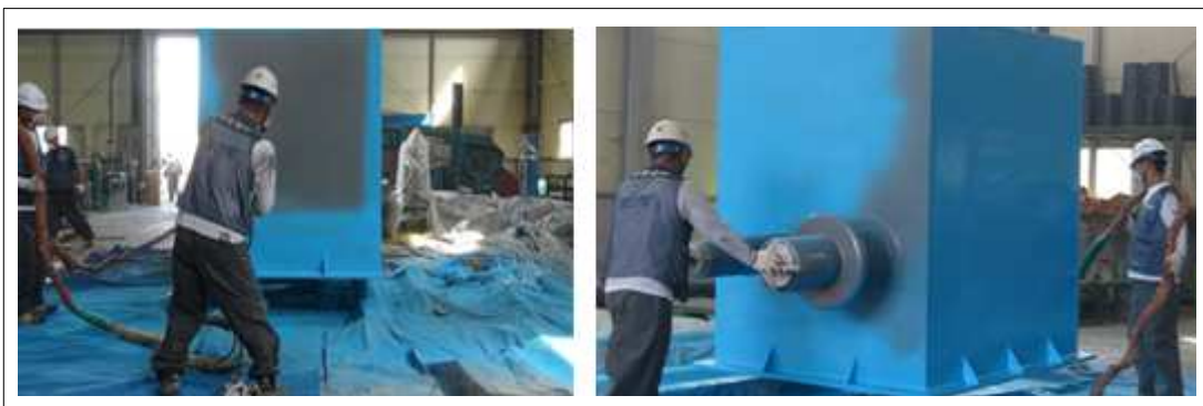
[KSC PU200 2nd 시공사진]
