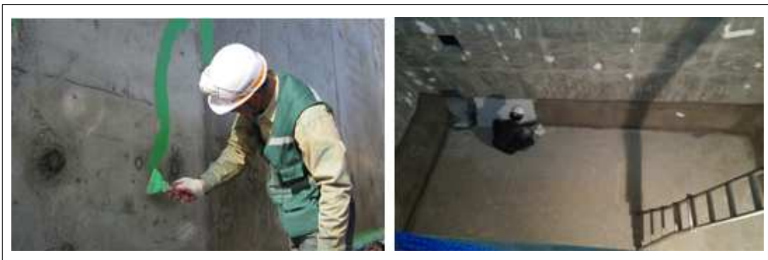
[KSC P100 1st 시공사진]
